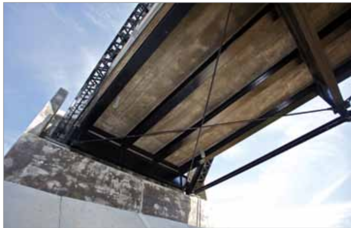
Below deck, stringers, sway bracing at abutment.
