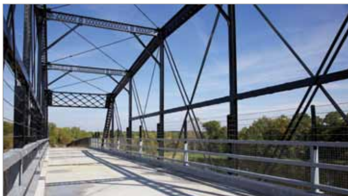
Cross bracing, verticals, diagonals and counters.
