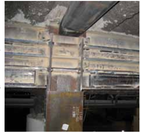
Figure 3: Typical drag retrofit connection.
