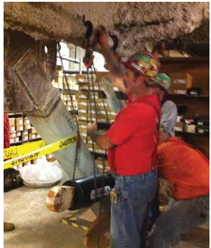
Figure 4: Installation of the viscous dampers by hand. Each damper weighs 500 pounds.
