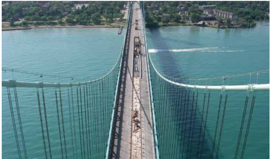
The rehabilitation of the suspended spans was performed in stages.
