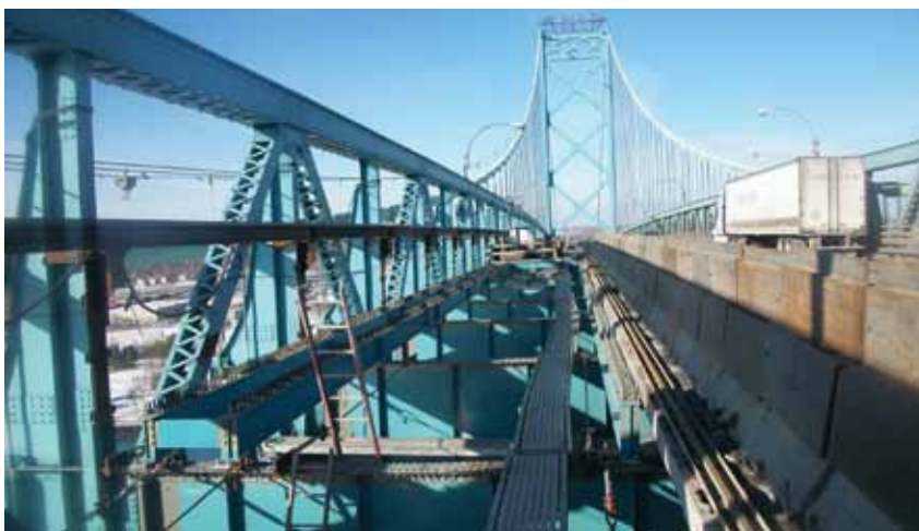
Staged construction was used to help maintain traffic.
