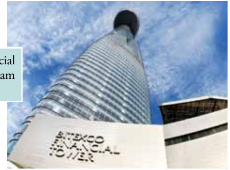
Bitexco Financial Tower rises above Saigon River, Ho Chi Minh City, Vietnam. Courtesy of the Bitexco Group.
