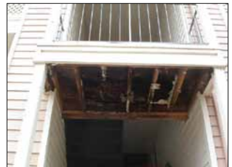
Figure 5: Breezeway with no plastic membrane installed.
