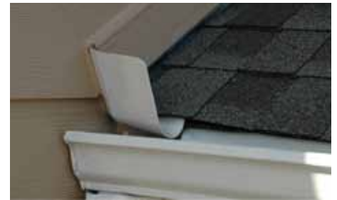
Figure 3: Kickout flashing.
