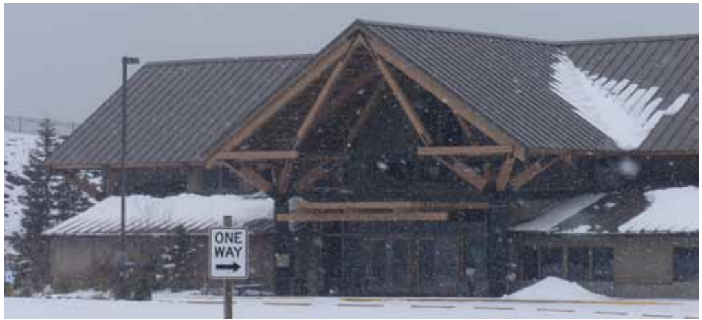
Figure 1: Sloped roof and overhangs protect the building from moisture accumulation.
