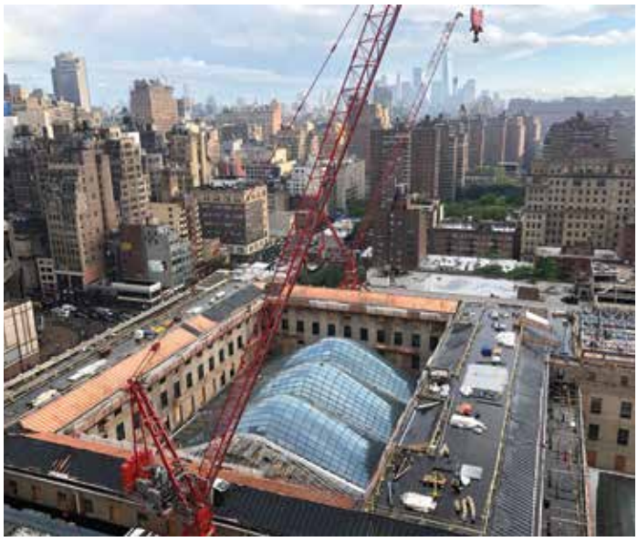
Main boarding concourse skylight installation.
