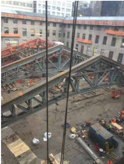
Existing trusses and reinforcement.
