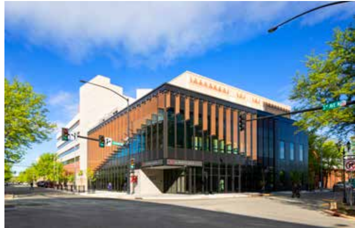
Cushing Terrell was an Outstanding Award Winner for the Alberta Bair Theater project in the 2021 Annual NCSEA Excellence in Structural Engineering Awards Program in the Category – Forensic/Renovation/Retrofit/Rehabilitation Structures under $20M.
