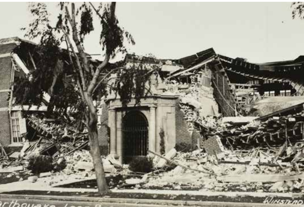
A school destroyed by the 1933 Long Beach earthquake.
