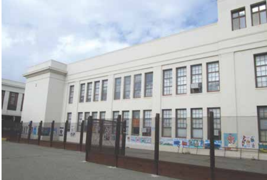
Structural debris fence surrounding an abandoned building.
