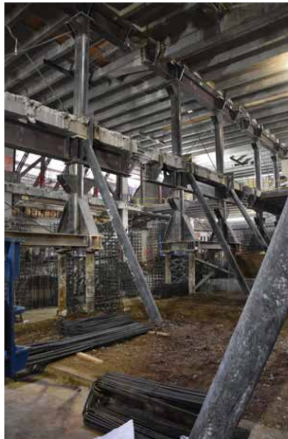
Figure 6. Shoring braced with the first floor demolished.
