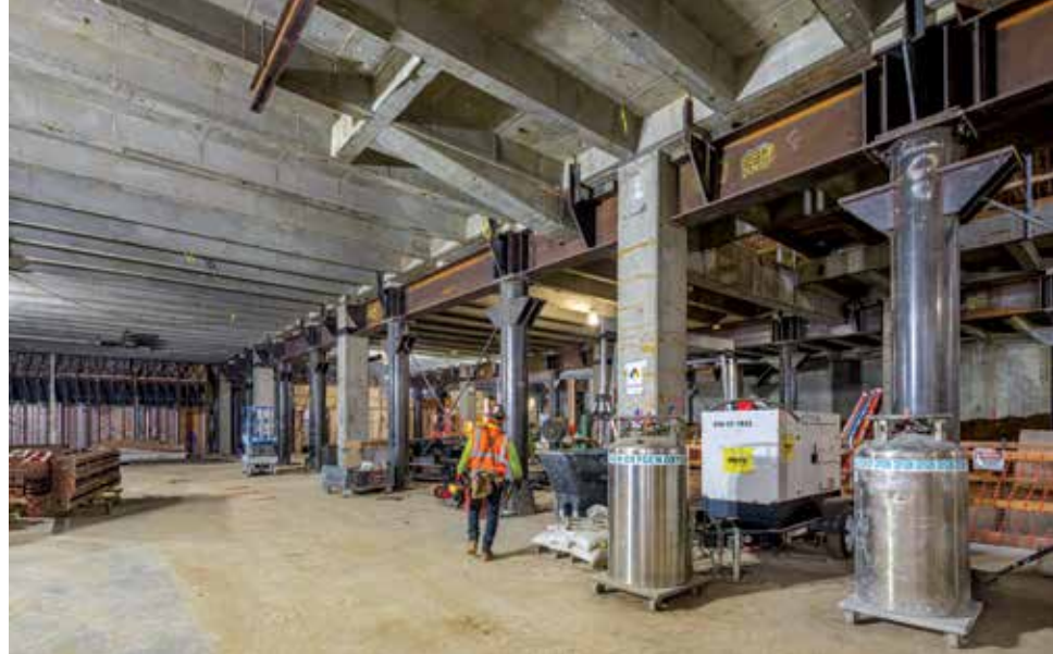
Figure 2. Completed shoring columns and beams prior to column demolition.
