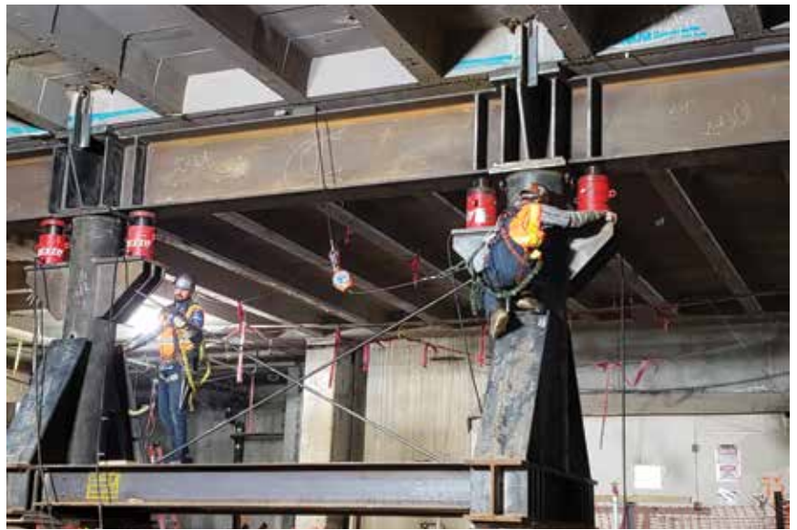
Figure 3. Setting up for test lift.
