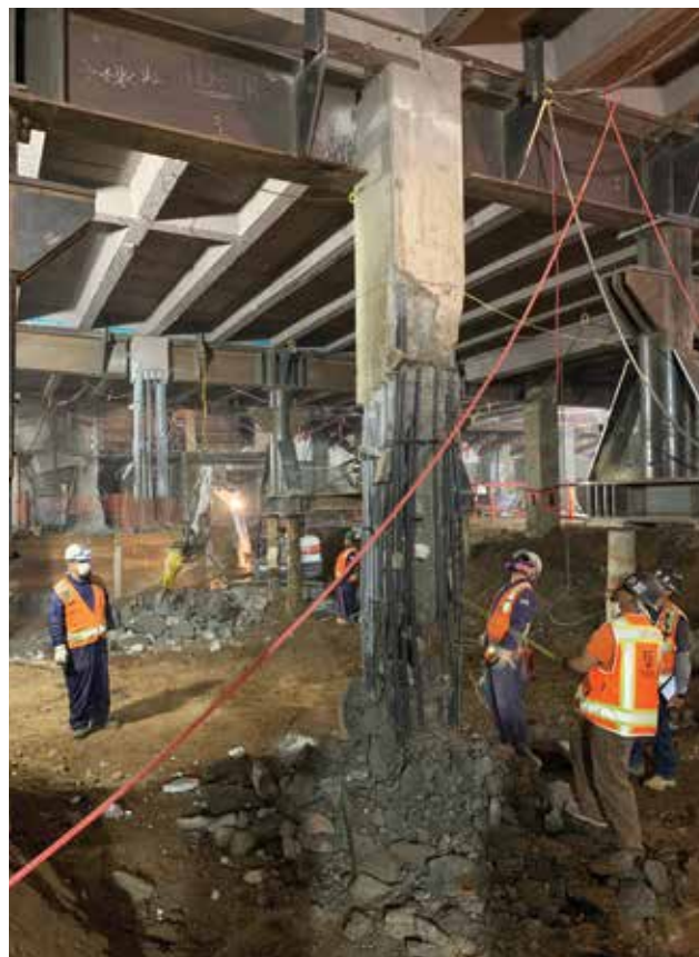
Figure 4. Column demolition with bars buckling.
