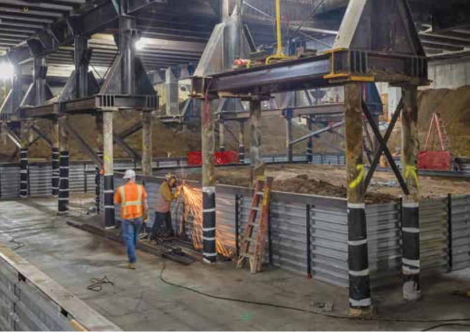
Figure 5. Steel foundation forms installed and building supported on exposed piles.
