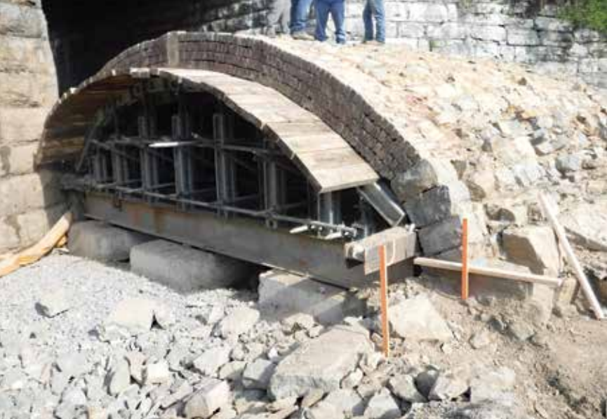
The East Burke Street Bridge arch as it is unearthed.
