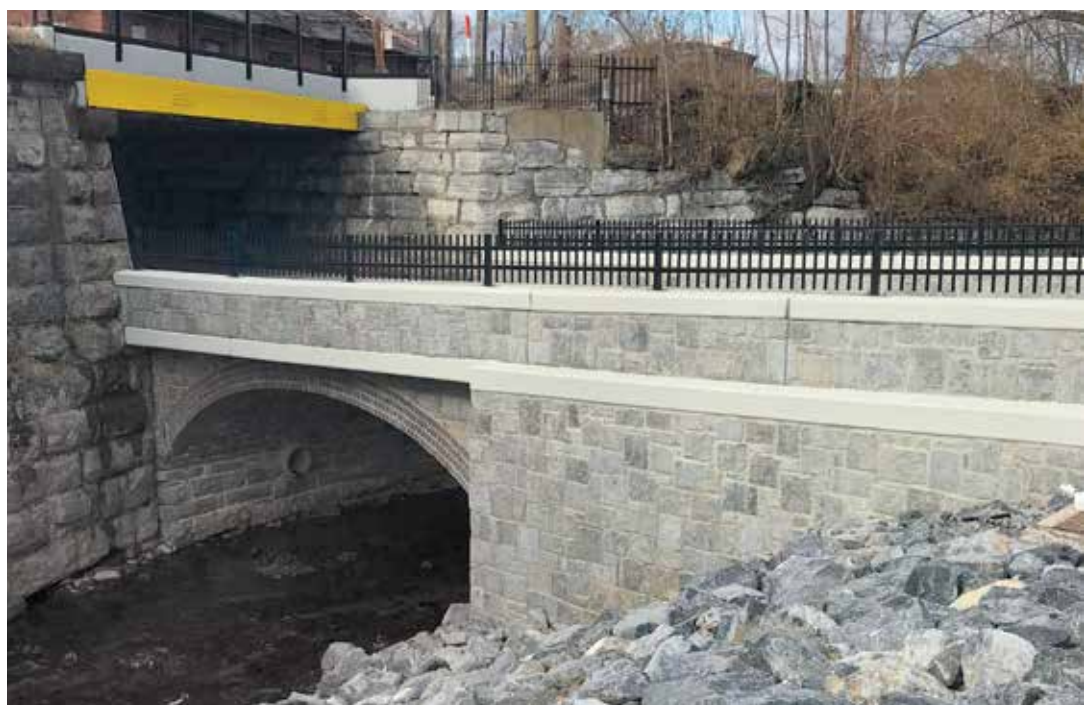
The East Burke Street Bridge following the renovation.
