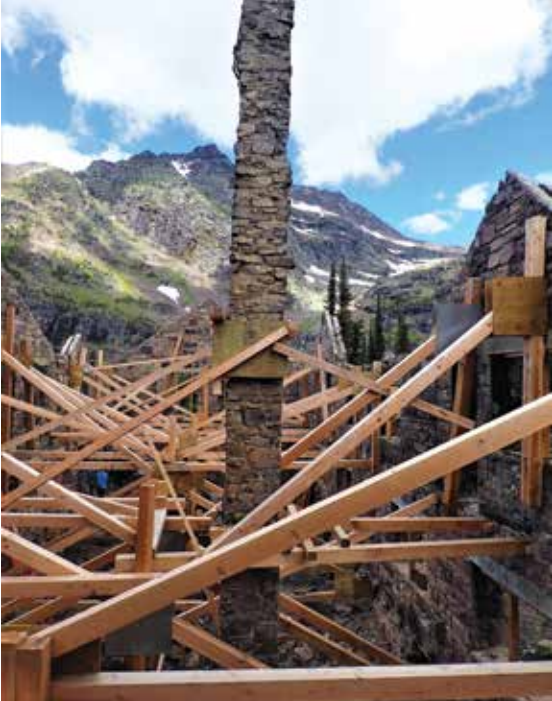
Figure 2. Designers assess the structure in July 2018 amongst the forest of braces.
