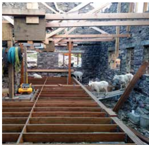
Figure 4. The first floor is framed as interior bracing is progressively removed.
