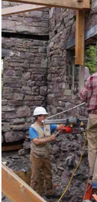
Figure 3. Engineers core-drill the masonry wall.
