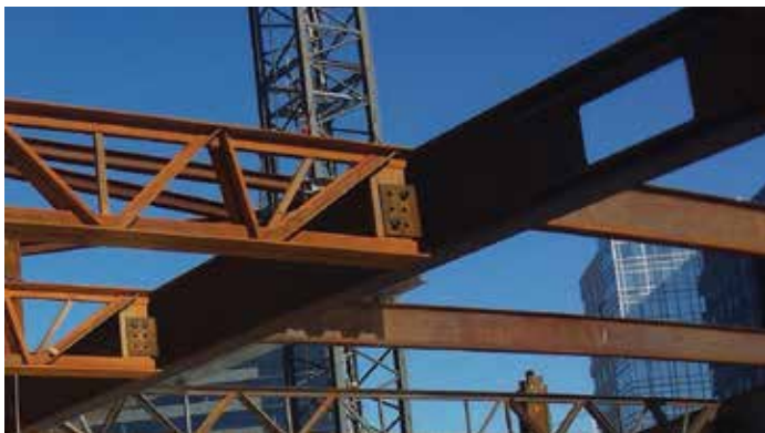
Bolted flush frame connections for joists to girder.
