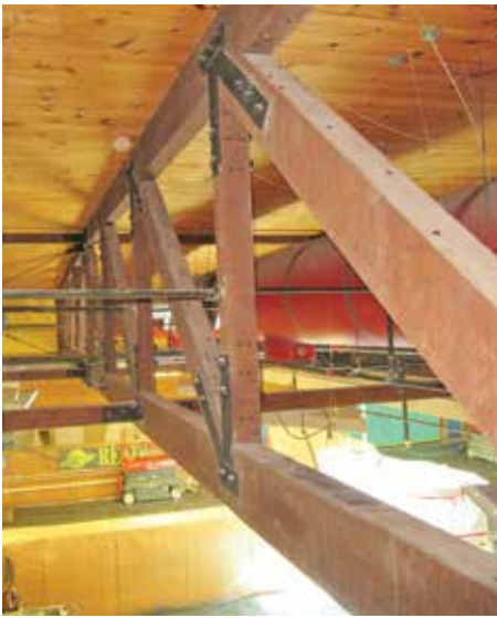
Repaired truss.
