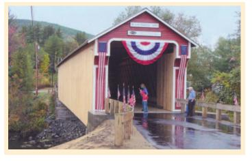
system, consisting of a small wire run through key portions of the bridge alerts the fire department. A deluge sprinkler and dry hydrant system were installed to allow the fire department to direct large amounts of water quickly to all portions of the bridge.
