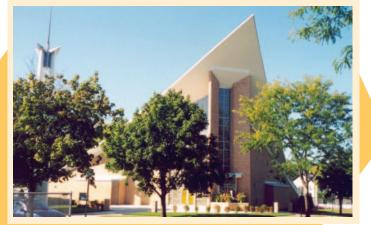
introduced and shell concrete beyond the edge beams was significantly thickened. The fin walls were laid up to the canopy soffit without mechanical attachment (i.e., the structure relied on friction to transfer shear forces).
