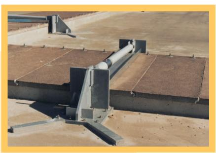
transfers the inertial load from slab to slab through the PSDs to the perimeter wall. The perimeter wall is loaded normal to its length, and the loads are then resisted by passive soil resistance.
