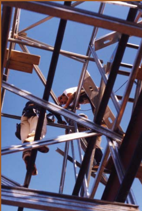
Truss bracing is an important element of both proprietary and c-shaped truss systems.
