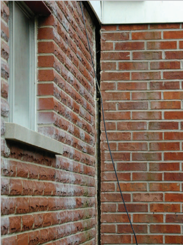
Foundation additional separation
