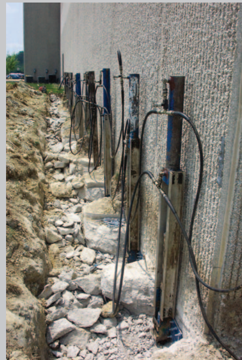
Commercial office building foundation stabilization
