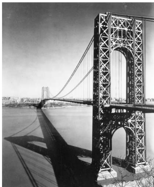
The George Washington Bridge began its service with a single-level roadway supported from below by a ribbon-like girder-truss. (Photographer unknown, courtesy of the Library of Congress)
