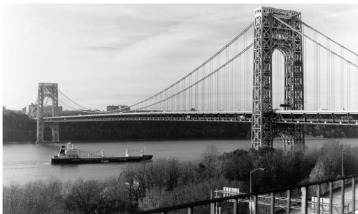
The George Washington Bridge after the completion of the lower deck in 1962. The bridge was designed for two decks, but only needed an upper deck during its first thirty years of service. (Photo, Jet Lowe; courtesy of the Library of Congress, HAER Collection)
