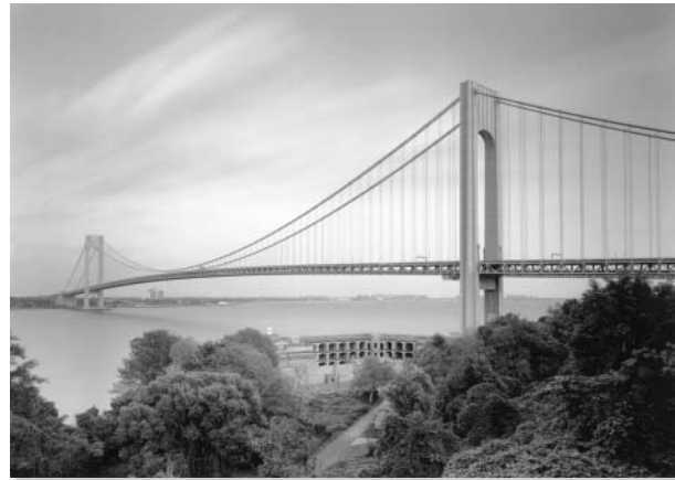
The Verrazano-Narrows Bridge. (Photo, Jet Lowe; courtesy of the Library of Congress, HAER Collection)
