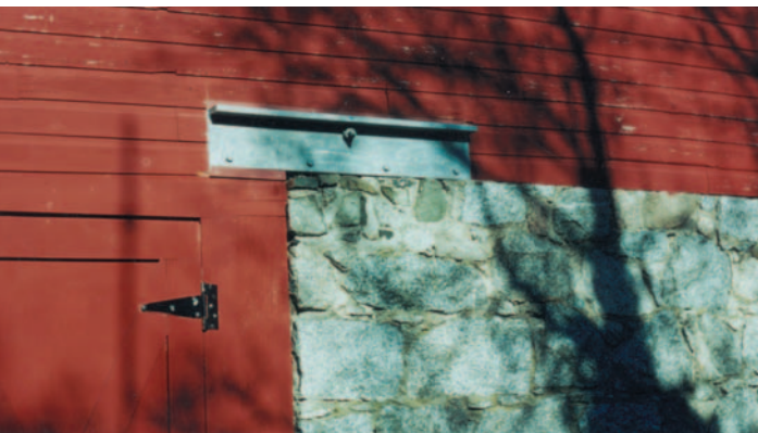
Load distribution angle at first floor
