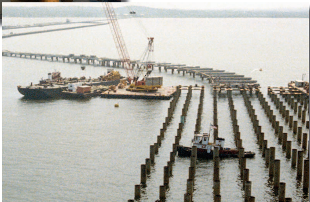
Figure 3: Floating Barges with “Ringer” Crane
