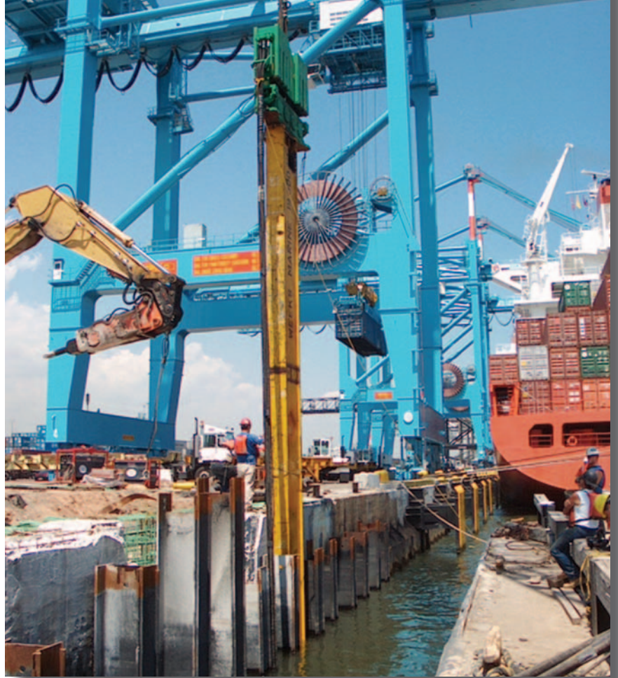
Figure 4: Driving of a King Pile System with a Vibratory Hammer
