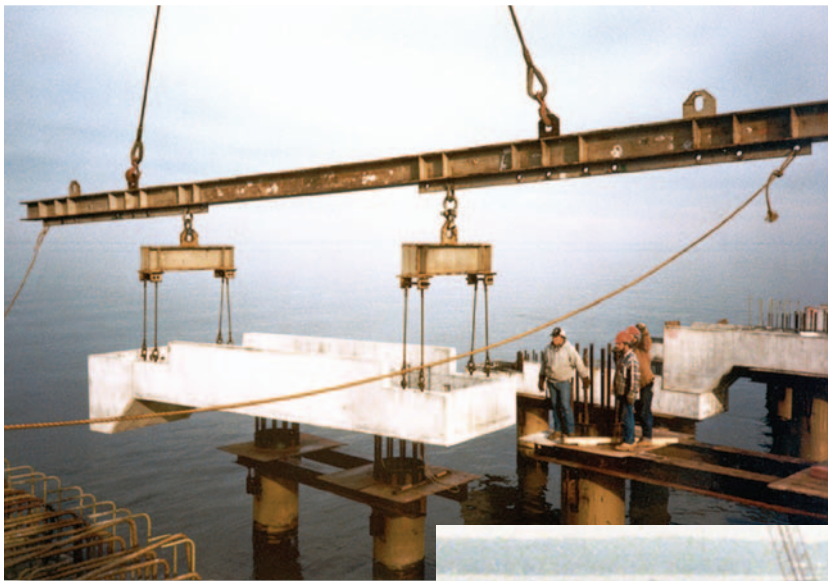
Figure 5: Installation of a Precast Pile Cap
