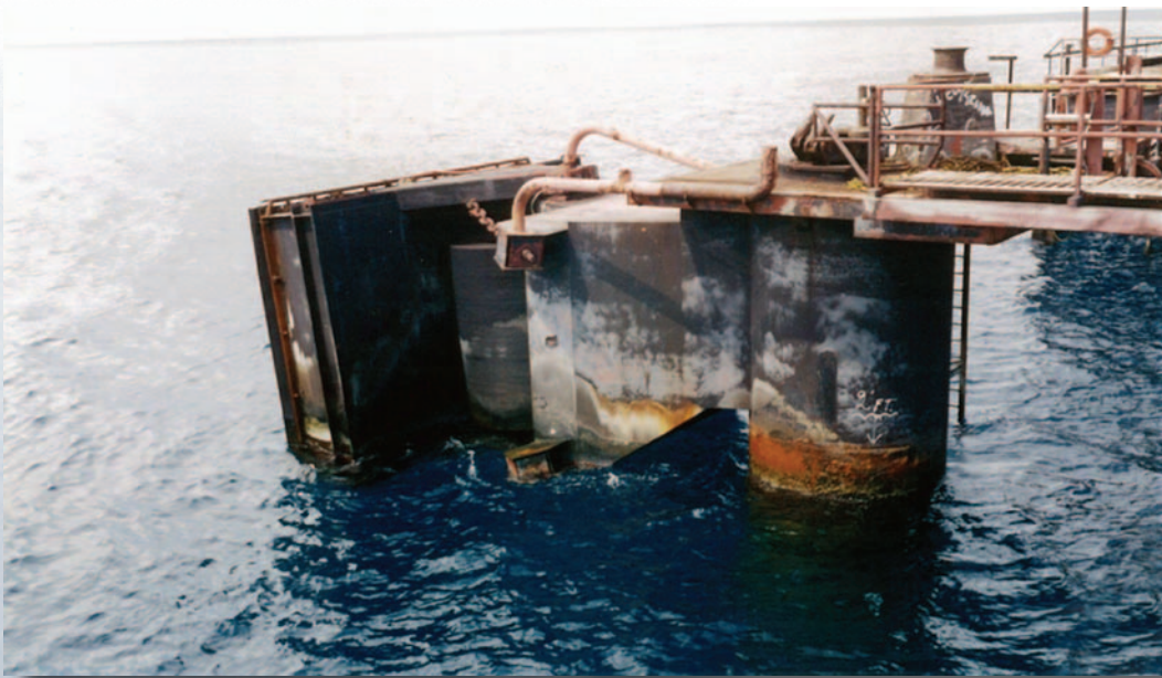
Figure 2: Monopile Type Breasting Dolphin
