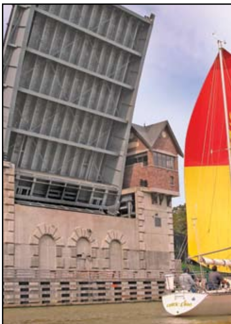
O'Rourke Bridge as a Sailboat Passes
