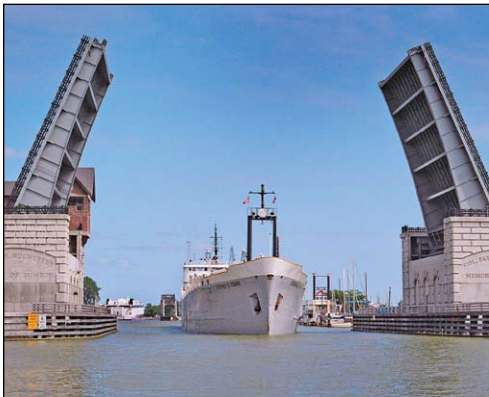
O'Rourke Bridge as Design Vessel is Passing Through
