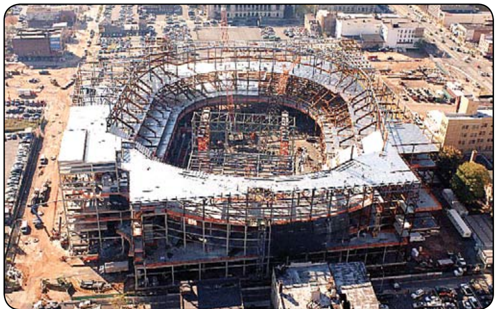
Figure 5: Aerial view of arena during construction
