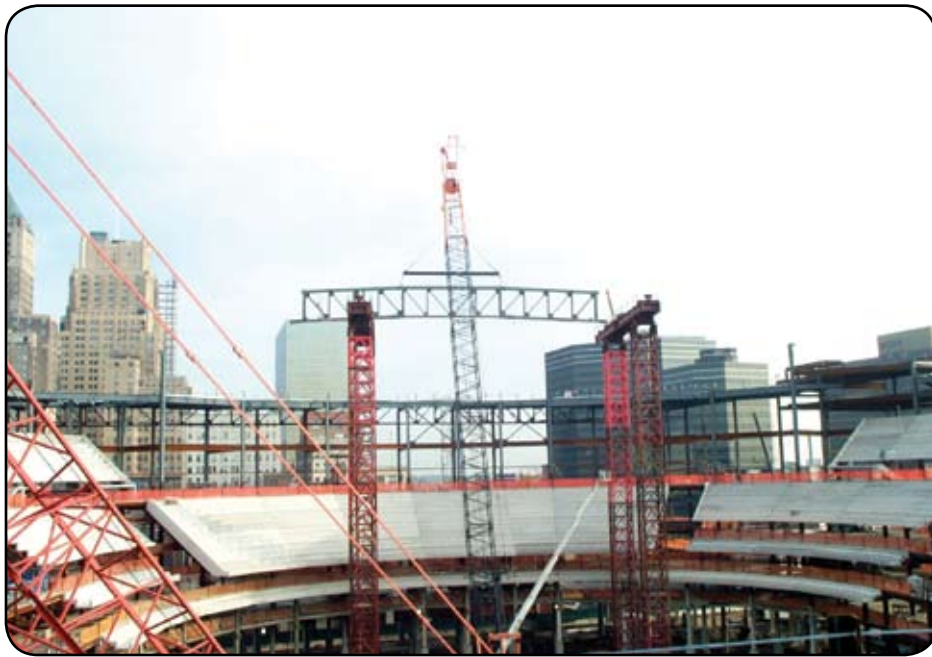
Figure 4: Roof Truss Erection
