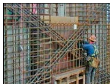
Figure 3: Typical diagonal reinforcement detailing in RC coupling beams (courtesy of Jack P. Moehle)
