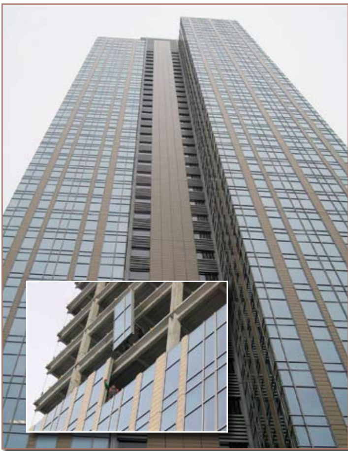
WAMU Center with vertical bands of panelized terra-cotta. Inset - WAMU unitized system under construction.
