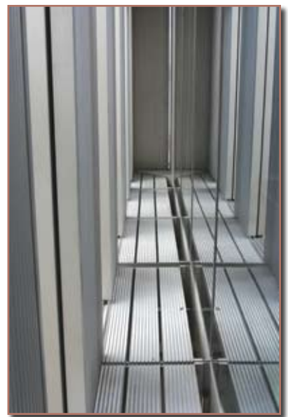
View of finished catwalk access zone.
