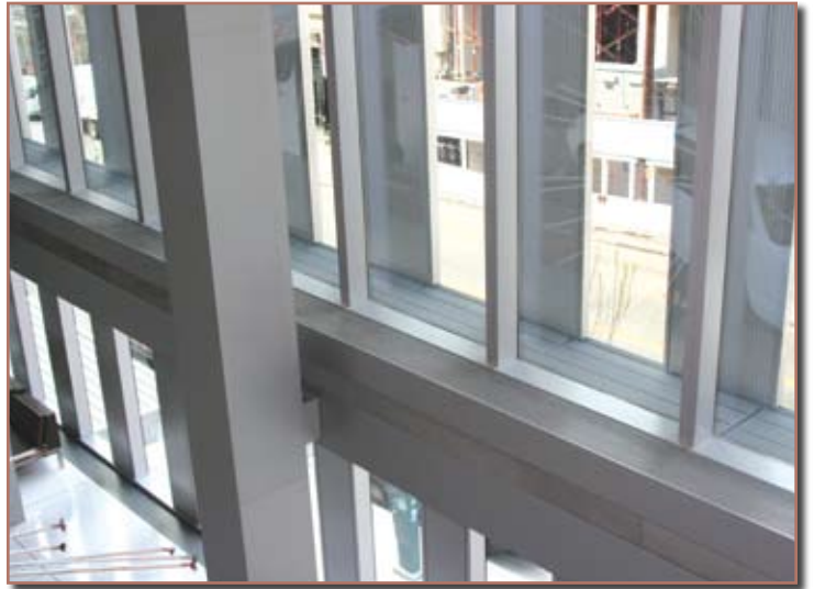
Interior view of multi-story gallery space with brise soleil partially closed.
