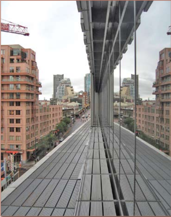
View from catwalk looking at tapered roof transition below during construction.
