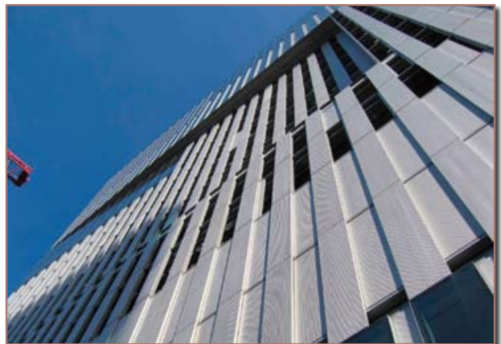
Lower 2 floors of brise soleil in closed position, upper floors fully open.
