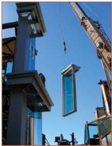
Glass unit with projecting catwalk being installed on SAM performance mock-up.
