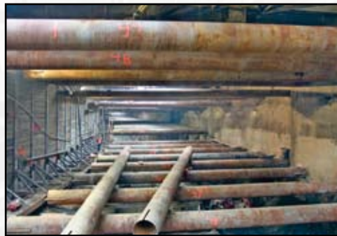
Tunnel excavation completed
