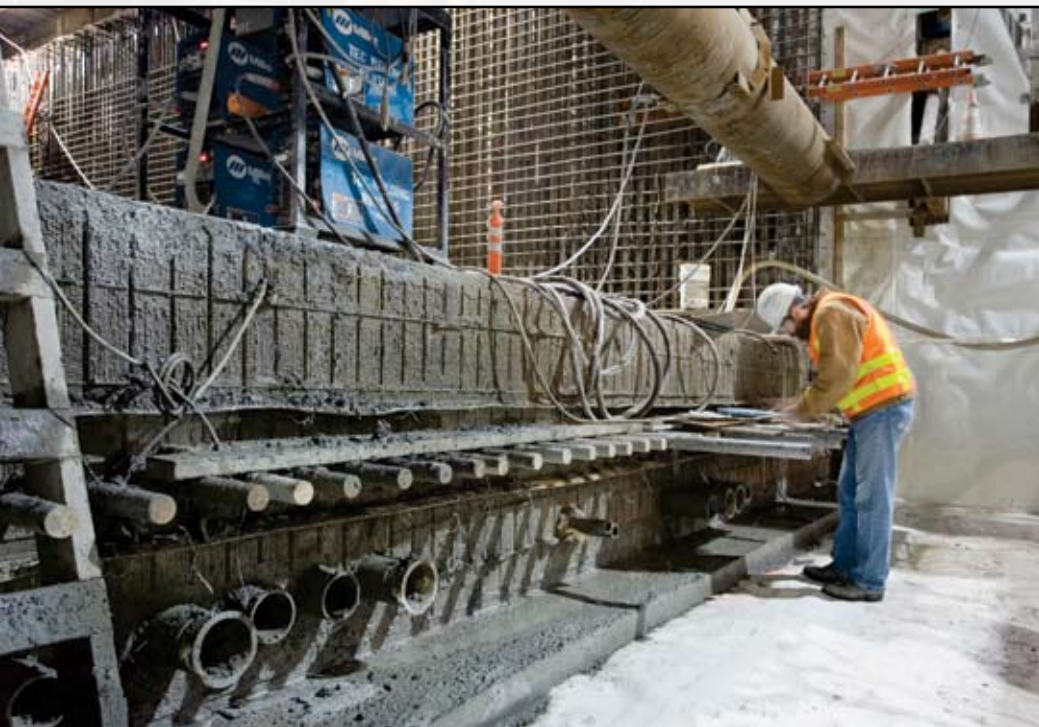
Tunnel base slab under construction
