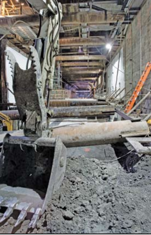
Tunnel excavation underway
