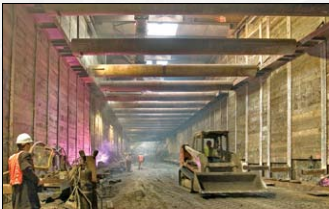
Tunnel excavation underway
