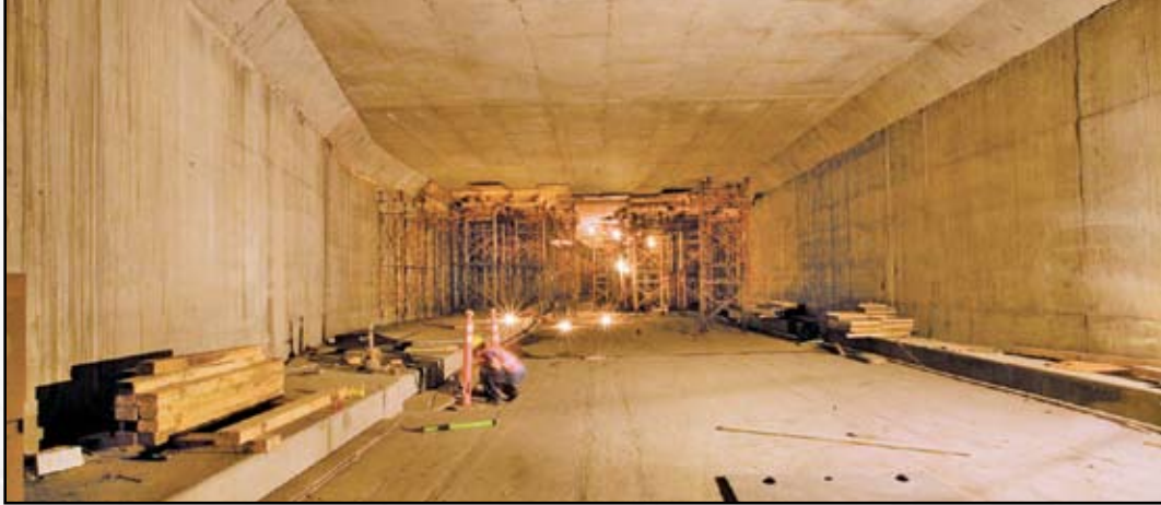
Completed tunnel segment
