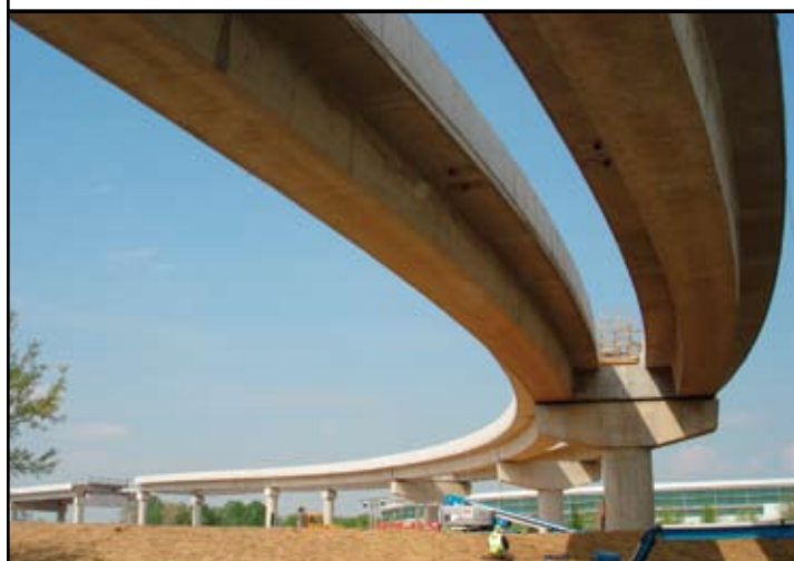
Figure 4: Cast-in-Place Girders.
