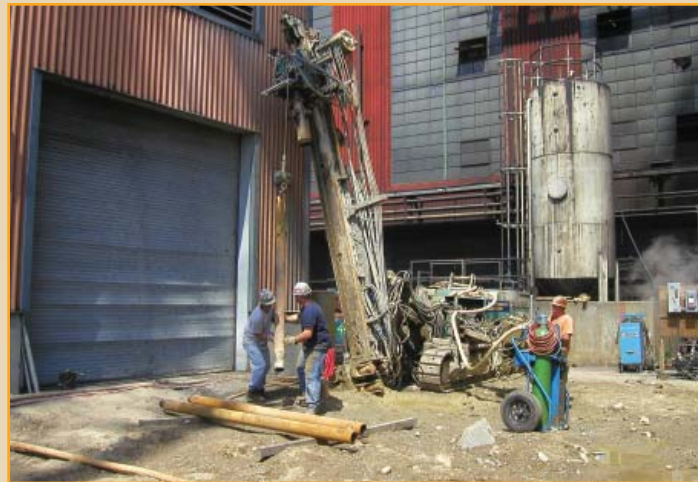
Figure 6: Hydraulic track drill installing battered micropiles
