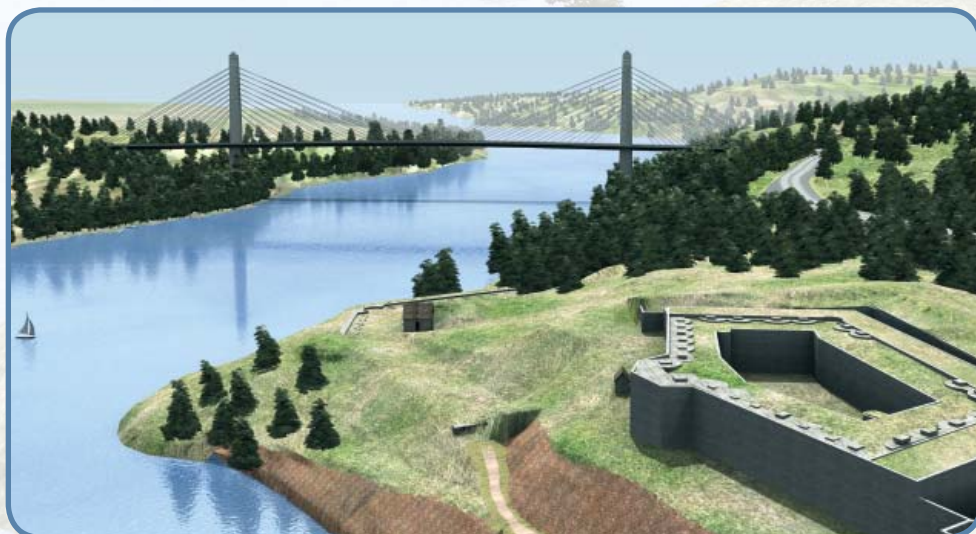
Rendering of the 1160 foot cable-stayed main span of the Penobscot River Bridge that will carry Route 1 along the Maine coastline and is located adjacent to historic Fort Knox near Bucksport, Maine. The western pylon will feature a multi-level observatory that will be open to the public.
