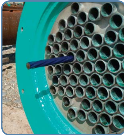
A "cheese plate" at each end of the cradle accommodates the individual strands for each cable stay. The stays range from 41 to 72 strands on the Penobscot River Bridge. FIGG holds U.S. Patent 6,880,193 on the cradle system.
