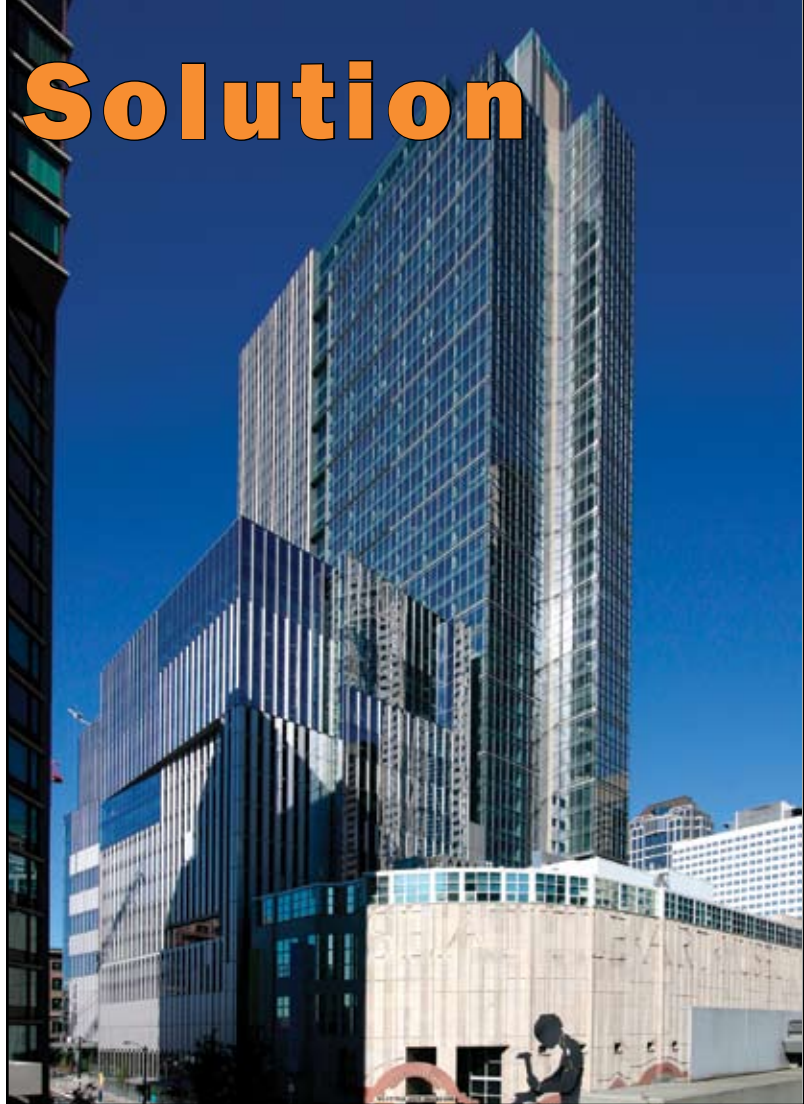
Figure 2: The new development features a 42-story, 540-foot-tall office tower and a 16-story, 240-foot-tall museum/office component. The two towers function as one structure but were designed to visually reflect the separate identities of the tenants, WaMu and SAM. Courtesy of Michael Dickter/MKA.
