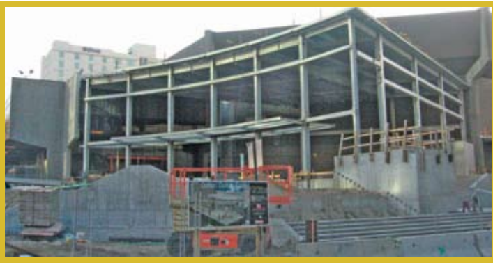
Figure 2: New main entry lobby at northeast corner of building under construction.
