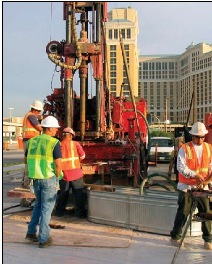
As part of the geotechnical exploration program, more than 125 borings were advanced to depths ranging from 25 to 250 BGS.
