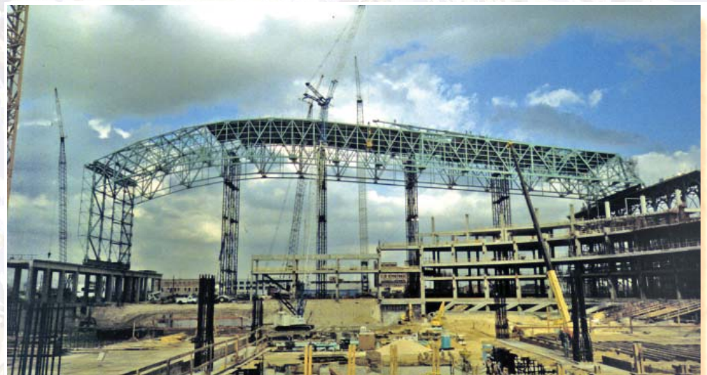
Figure 2: Erection Towers for Minute Maid Park, Houston, Texas. (photo by Mark Scheyer)
