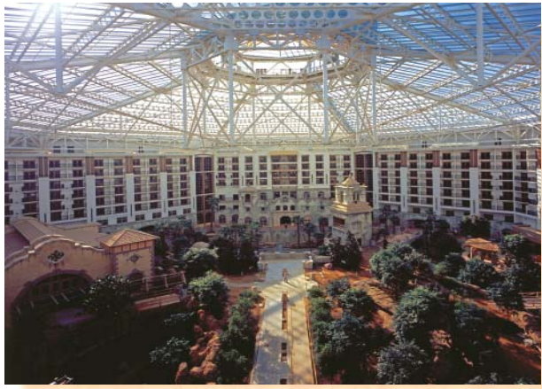
Figure 3: Gaylord Texan Resort and Convention Center, Grapevine, Texas. (photo by Dallas Visual Design)
