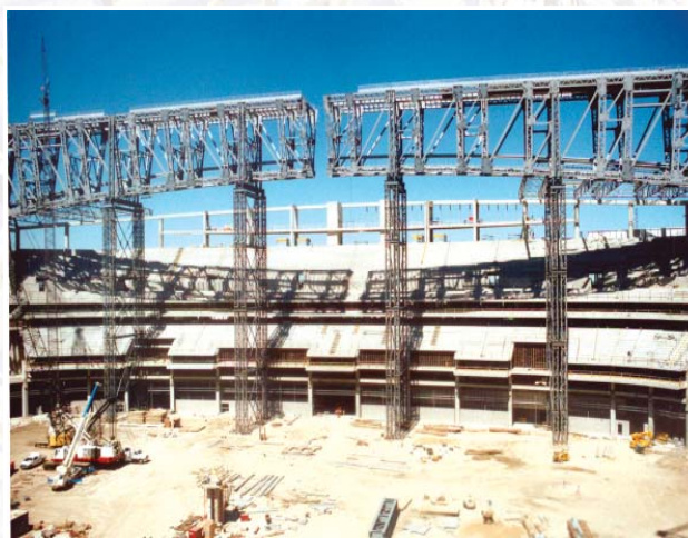
Figure 6: Erection of the Supertruss, Reliant Stadium, Houston, Texas.
