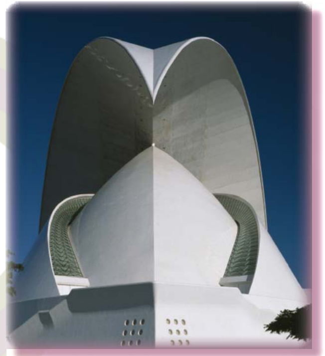
The stunning, wave-like roof of the Auditorio de Tenerife (2003), in the Canary Islands, designed by Santiago Calatrava, exemplifies the sculptural possibilities of reinforced concrete. Photo by Alan Karchmer for Santiago Calatrava
