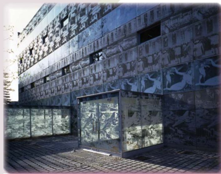
The Library at the Eberswalde Technical School (1999), in Eberswalde, Germany, by Herzog & de Meuron, uses photoengraved concrete. Image © Margherita Spiluttini
