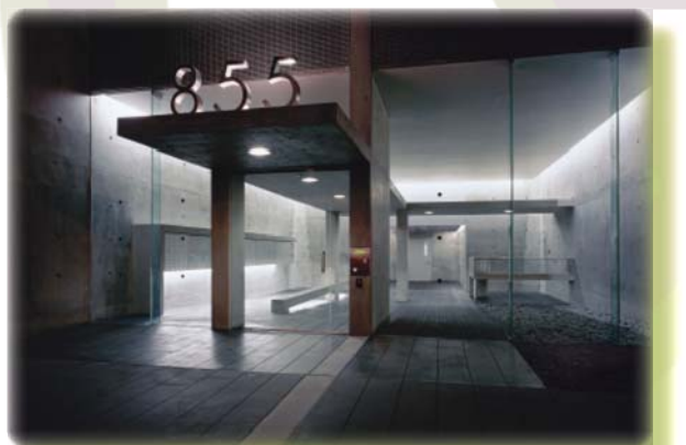
Yerba Buena Lofts (2002); San Francisco, CA: Stanley Saitowitz Office/Natoma Architects, Inc. Photo © Tim Griffith
