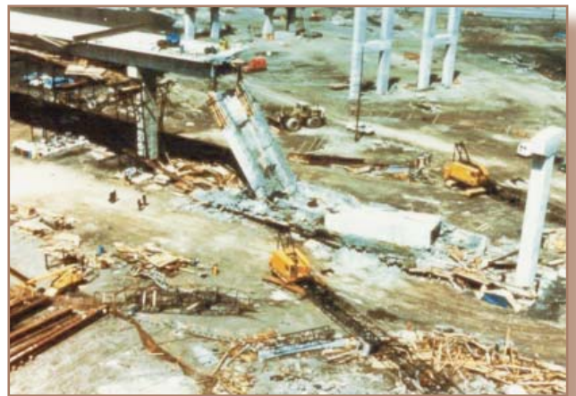
Cline Avenue Overpass failure, Chicago, IL (1982).
