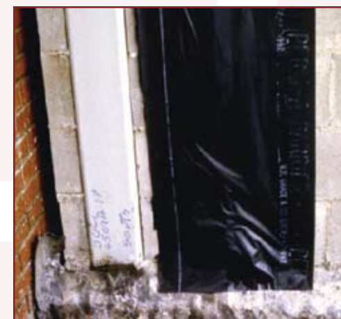
Figure 3B: Column and spaces are protected by membrane flashing
