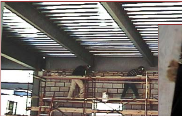
Figure 16: Grouting bond beams too close to the bottom of steel beams can be difficult
