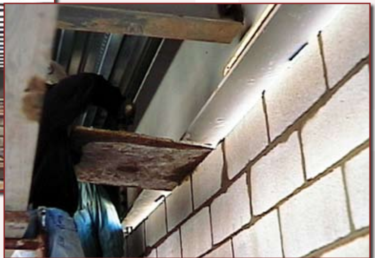
Figure 16: Grouting bond beams too close to the bottom of steel beams can be difficult
