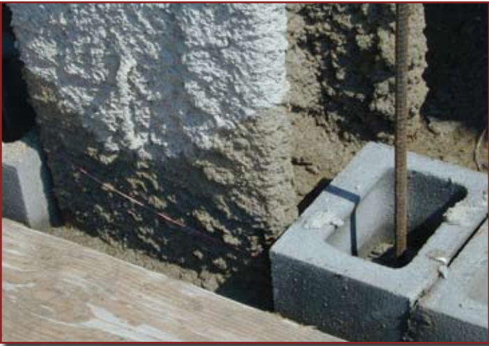
Figure 9: Columns with fireproofing or voids
