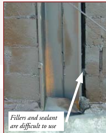
Figure 3A: Unprotected column
