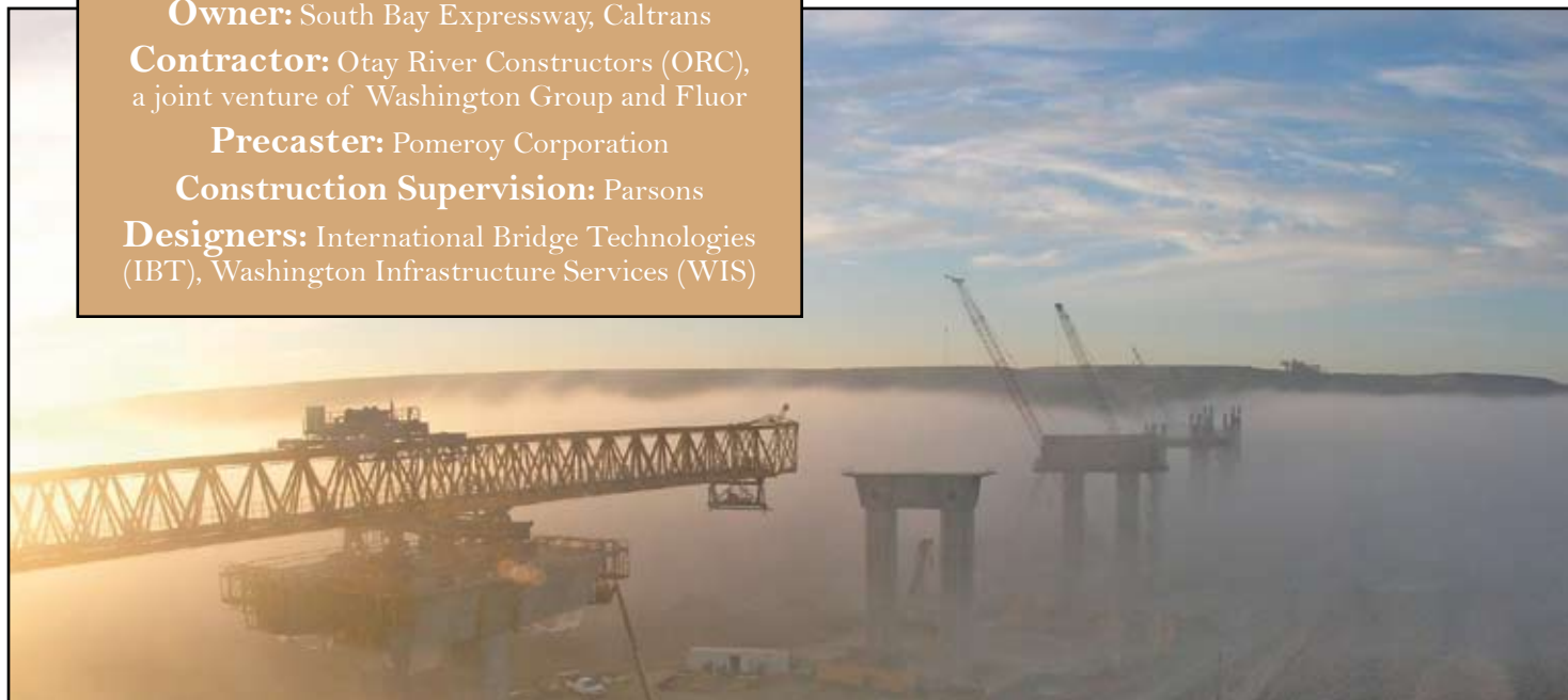
Dawn breaks as construction gets underway on the Otay River Bridge.
