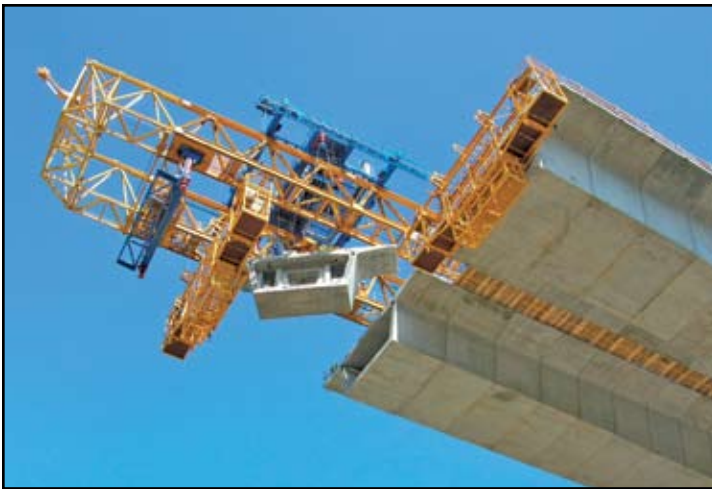
A segment is swung into position at the cantilever tip.
