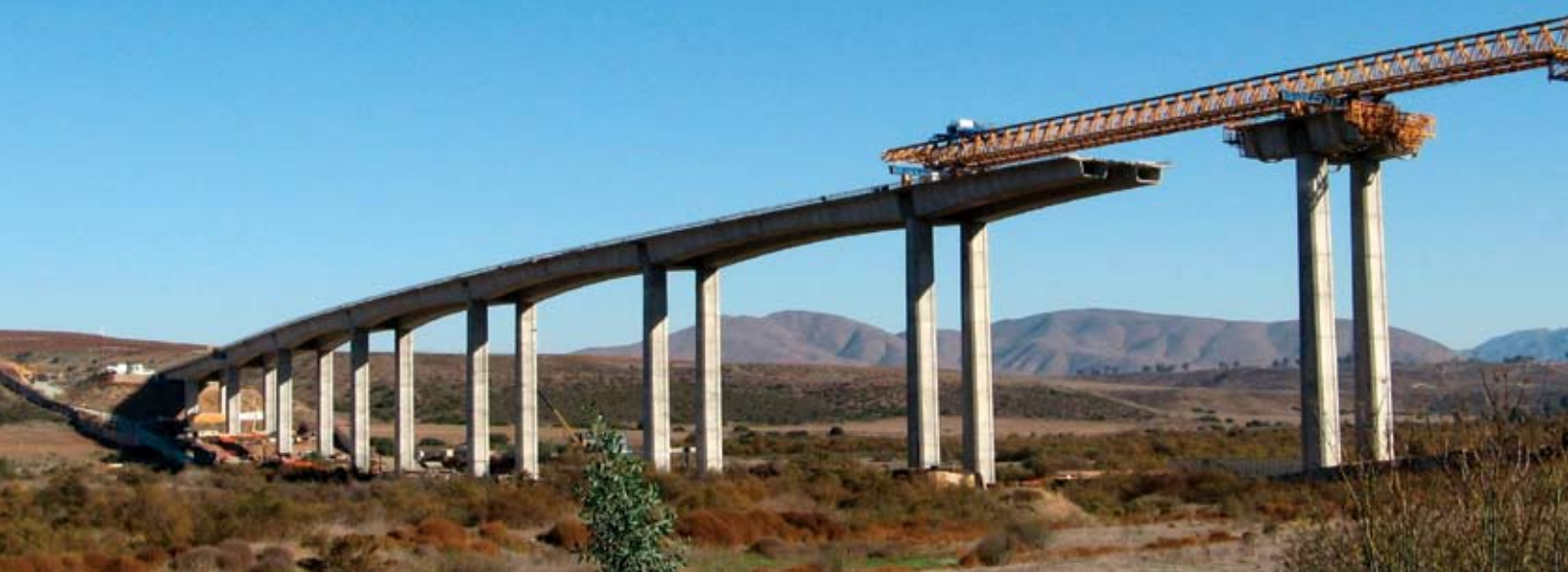
Segments are delivered via an overhead gantry, eliminating the need for falsework.
