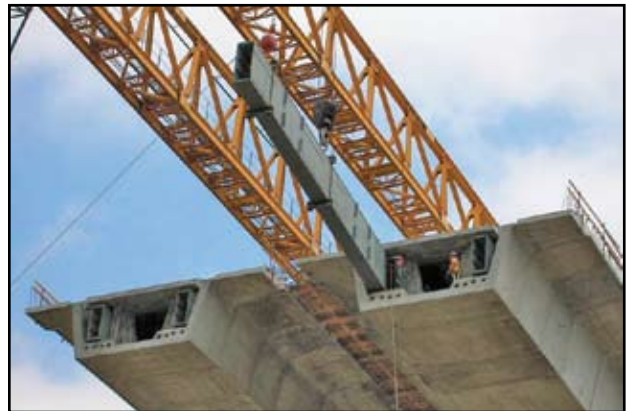
Steel beams are installed for the mid-span expansion joint.
