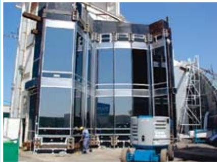
Figure 6a: Tower Test Mock-up Assembly.
