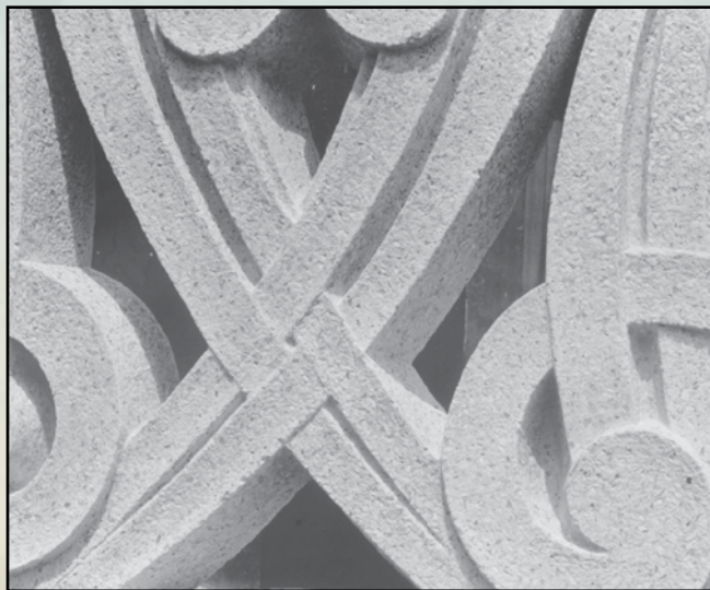
The darker spots are the translucent quartz and the white spots are the opaque quartz
