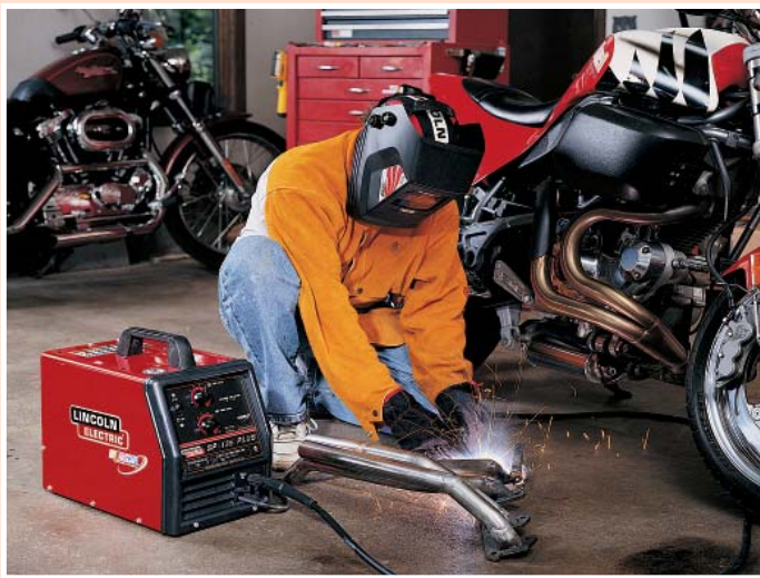
Figure 3: Small, portable 120 volt wire feeder/power source combinations may look lightweight, but when produced by a reputable welding manufacturer, they can be ideally suited for welding on gage materials—even for structural applications.
