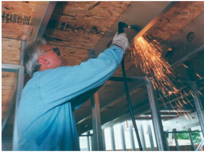
Figure 5: Plasma arc cutting provides for fast, quality cuts on sheet steel, something that is nearly impossible with oxy-fuel cutting. Additionally, plasma cutting can be used to cut nearly any electrically conductive material, including stainless steel and aluminum.
