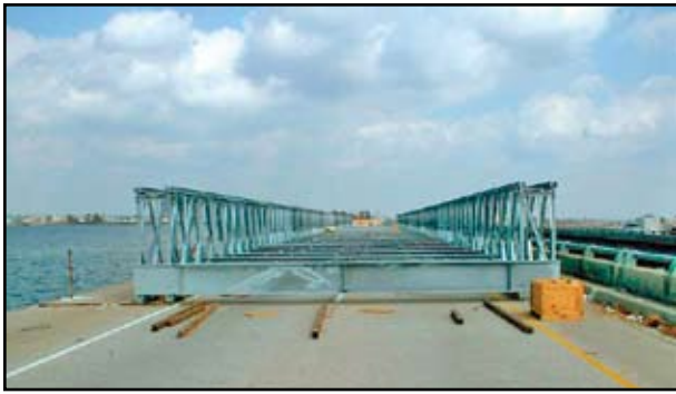
Figure 3: Temporary Acrow Span for the WB Bridge
