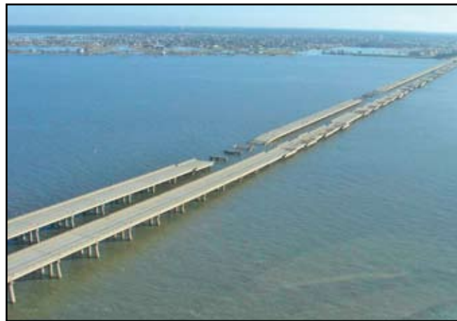
Figure 1: Damaged I-10 "Twin Spans" looking north
