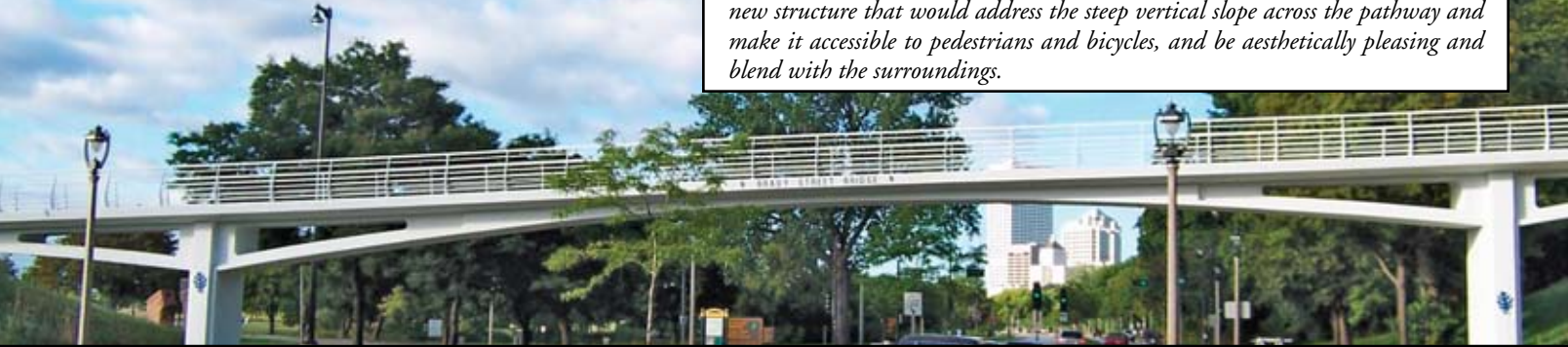
Brady Street Bridge Looking South.
