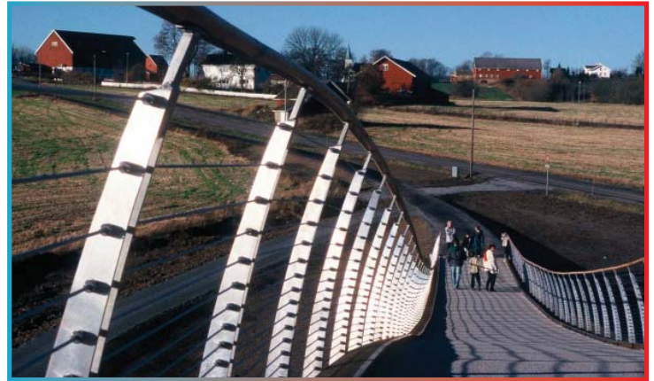
Pedestrians exiting at the west end, after crossing over the bridge.
