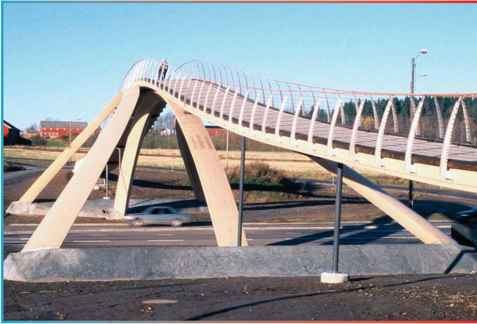
View showing the slender steel pipe pillars (columns) that support the pedestrian pathway from the arched timber structure, which spans the motorway, to the terminus of the deck at ground level. Also, evident is the detailing of a splice connection in the main vertical arch.
