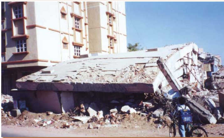
Figure 1. Earthquake reconnaissance observations from India showing structural systems that did and did not perform well.
