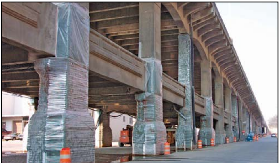
Several piers undergoing ECE treatment process. Courtesy of Vector Corrosion Technologies.
