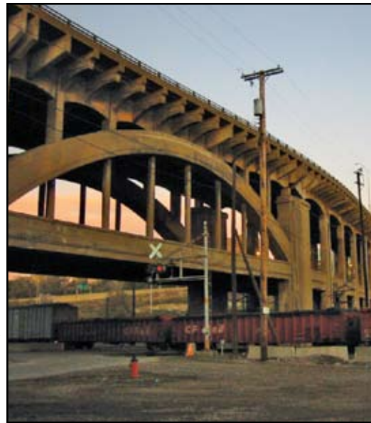
12 th Street Viaduct, 2005. Courtesy of Vector Corrosion Technologies.
