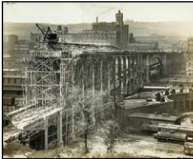
12 th Street Viaduct Under Construction, completed in 1915. Courtesy of HNTB Corporation and Architectural & Historical Research Consultants.
