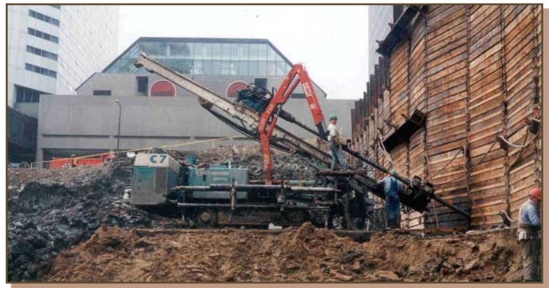
Tiebacks for anchored temporary wall being installed as excavation progresses
