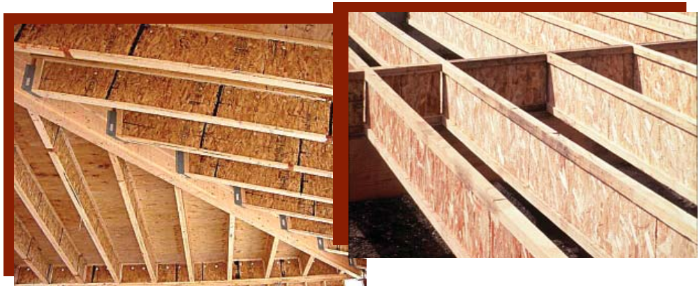
I-Joists used in roof-framing applications
