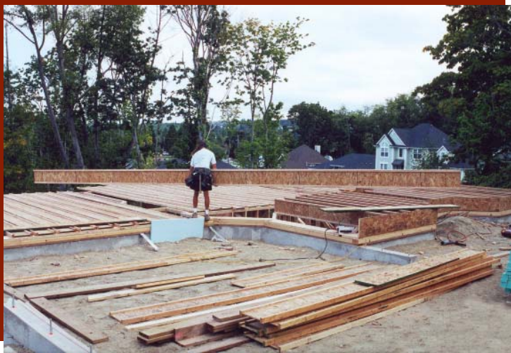
I-joist are light wieght and easy to handle on the job-site
