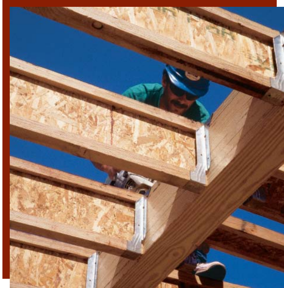
Hangers designed specifically to accommodate I-Joists
