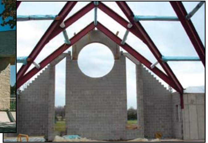
Chapel under construction showing loadbearing masonry walls.
