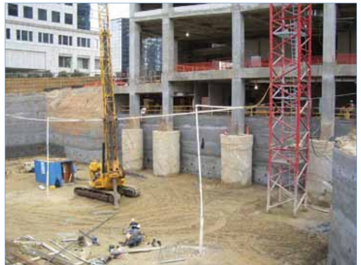
Combined Tower Column/Drilled Pier.
