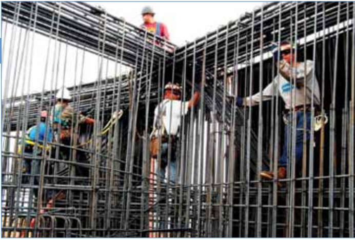
Transfer Beam Construction.
