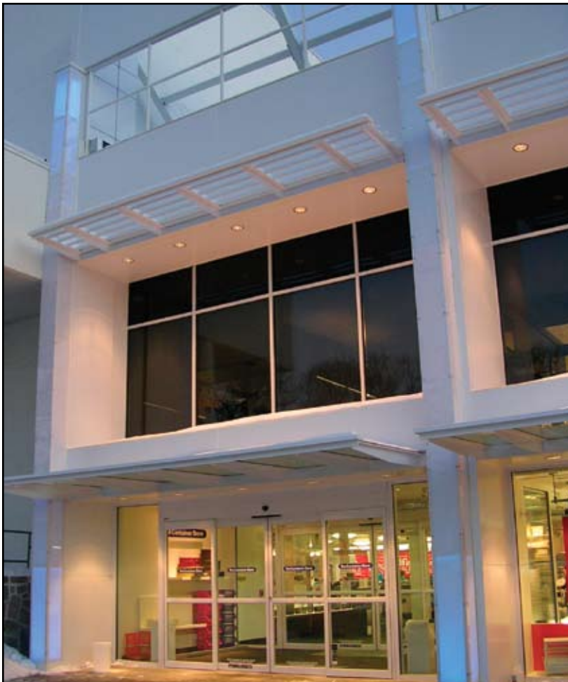
View of finished product entrance to the store.
