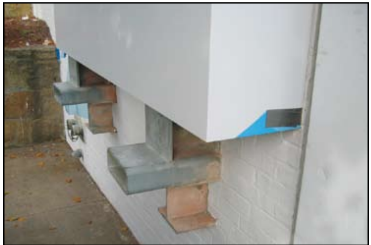
Cantilever extension support at base.
