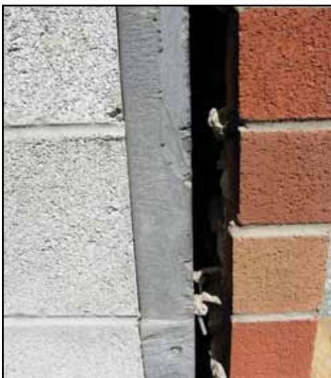
Figure 5: Brick and concrete masonry wall under construction.
