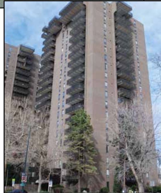
Figure 6: High rise load-bearing brick building, Park Lane Towers, Denver, CO. Courtesy of Diane Travis, Rocky Mountain Masonry Institute.
