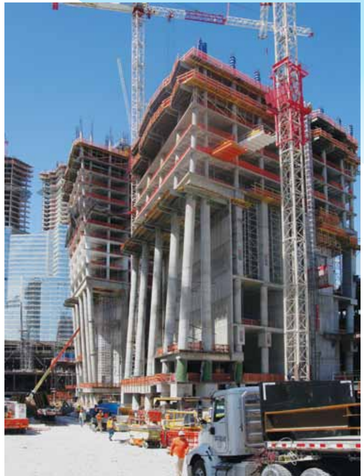
Figure 2: South Façade Inclined Composite Lobby Columns under Construction.
